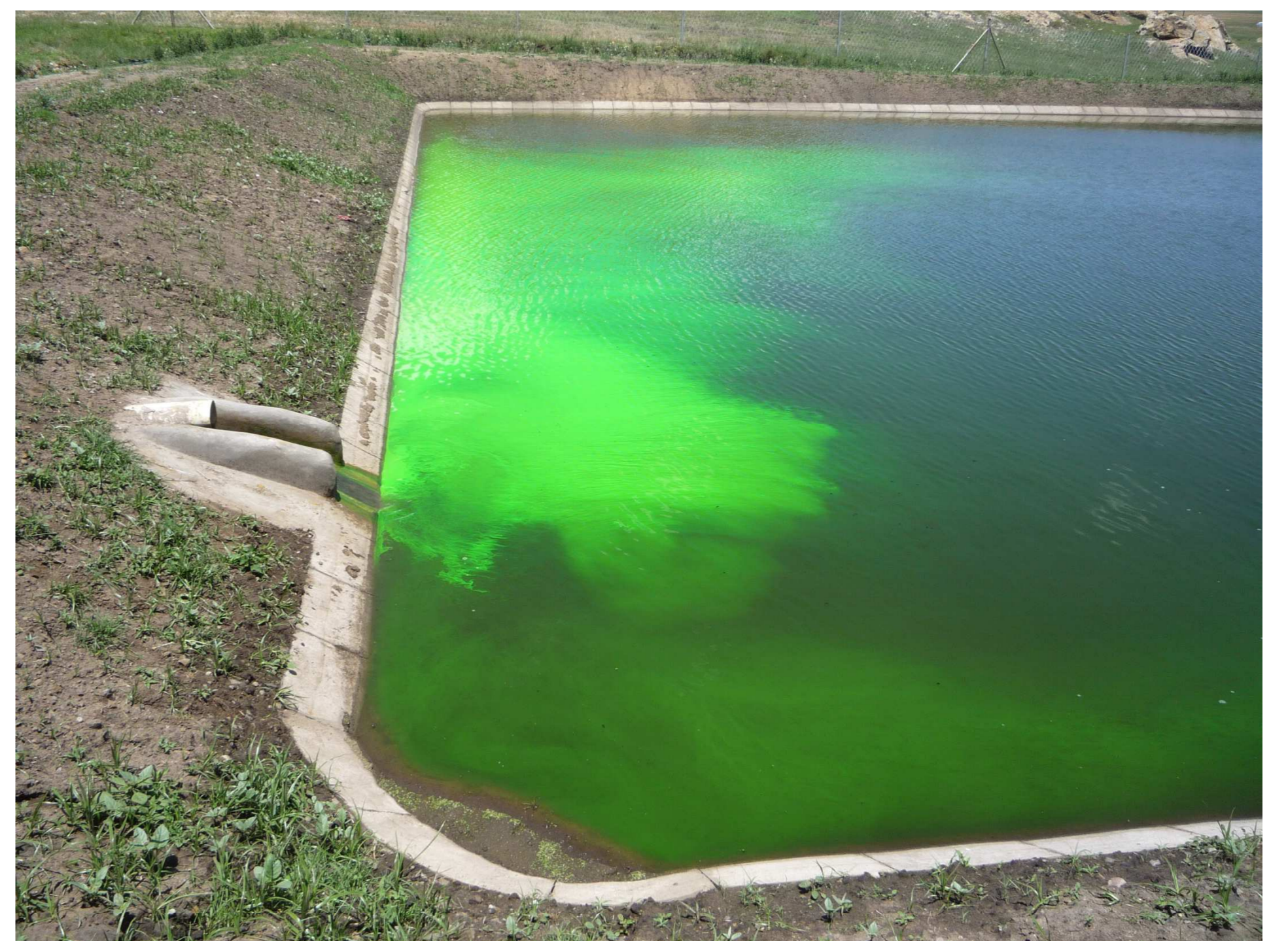
Picture 1: Tracer test at maturation pond in HA NYENYE
