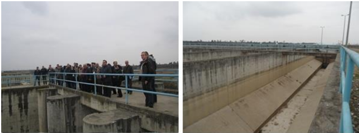
Ganjafrooz diversion dam
